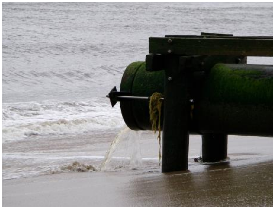
Storm water outfall.
